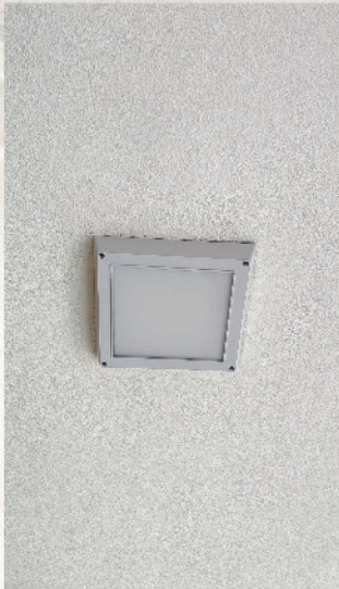
1. Installing LED lights
