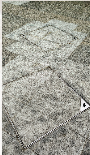
2. Replacing the drainage lids
